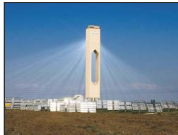
Figure 8: A power plant in Spain, which uses energy from the Sun, instead of coal, to produce the steam that runs its generators. Because of the dust in the air, one can actually see the path of the Sun's rays. Acknowledgment: http://en.wikipedia.org/wiki/PS10_solar_power_plant#/media/File:PS10_solar_power_tower.jpg
