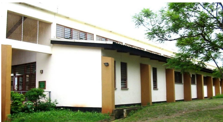
Part of Bunda College Library Building
